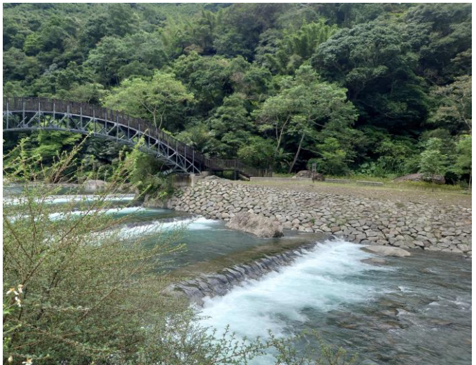
Groundsill works and bank protection
